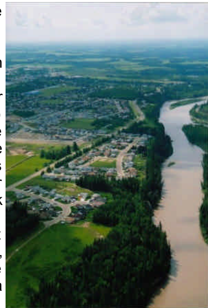
The town of Rocky Mountain House today.
